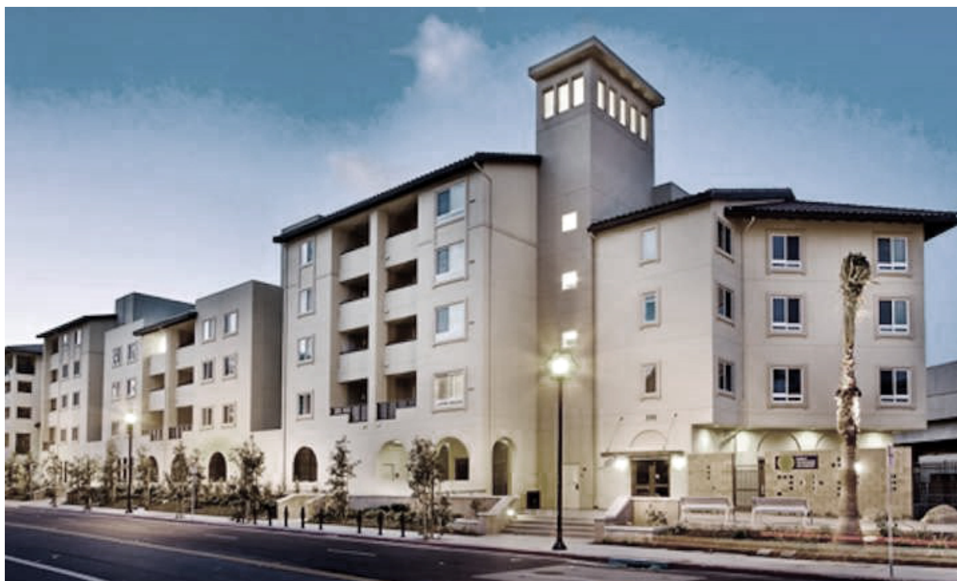
Social housing project "Trestle Glen" just south of San Francisco, credit: www.bridgehousing.com
